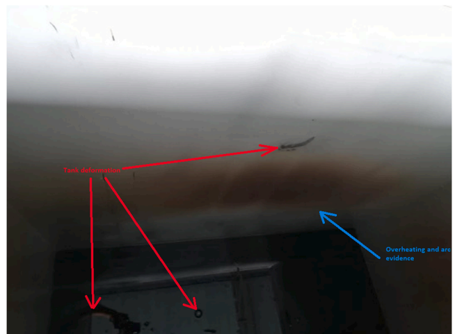
Fig. 12. deformation of the tank's side walls and several discharge points.
